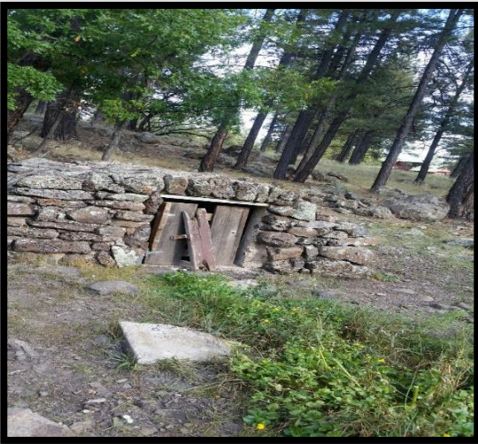
Figure 1- Spring box flow in fall 2015
